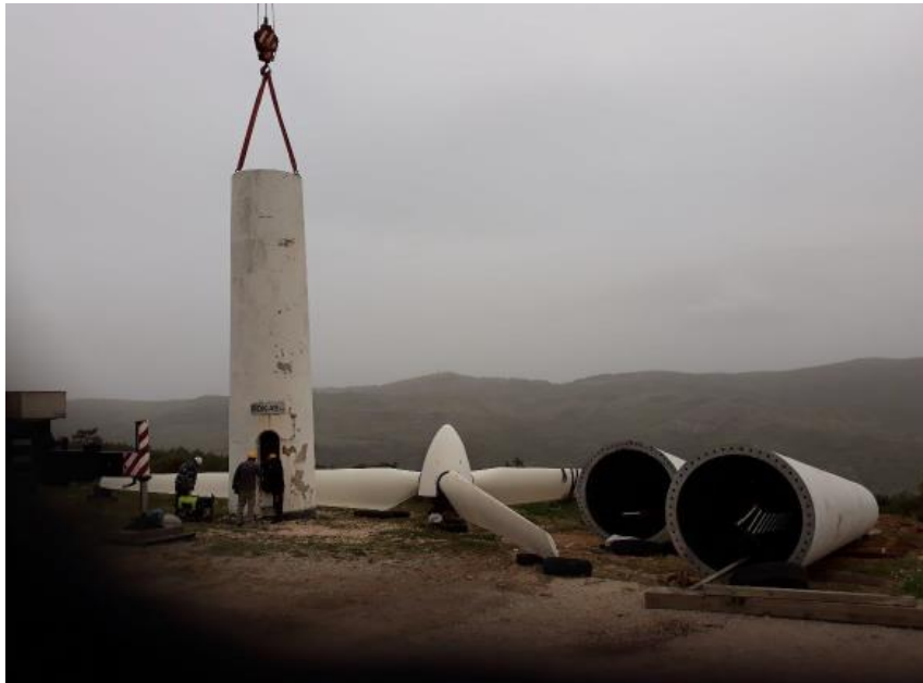
Dismantling of a G/G pillar (PPC renewable project)
